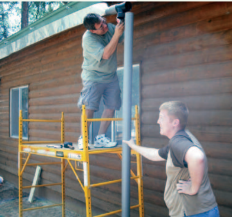
Gutter and Downspout Installation
